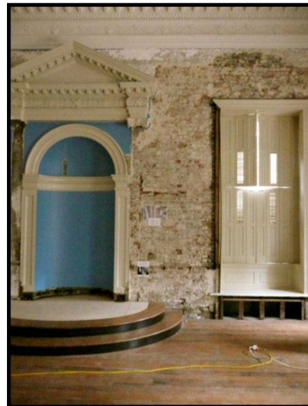
After: 2008 removal of top riser achieves a dais closer to original proportions, including a broader landing
