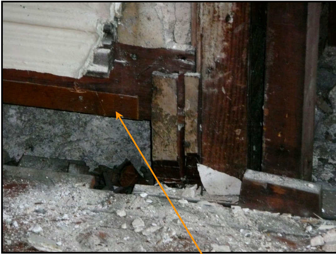
Reused board with 1878 maple graining
