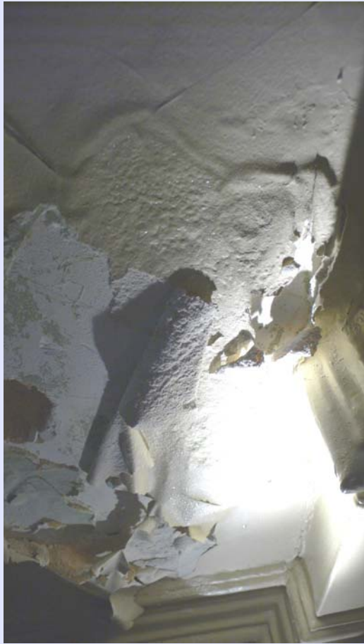
Liquid water condensed on the surface of the plaster in the corner of the Old Senate Chamber and running down the wall.
