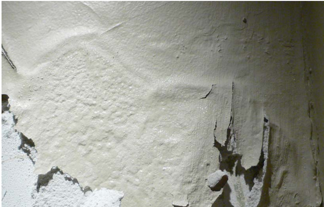
Liquid water condensed on the surface of the plaster in the corner of the Old Senate Chamber and running down the wall.
