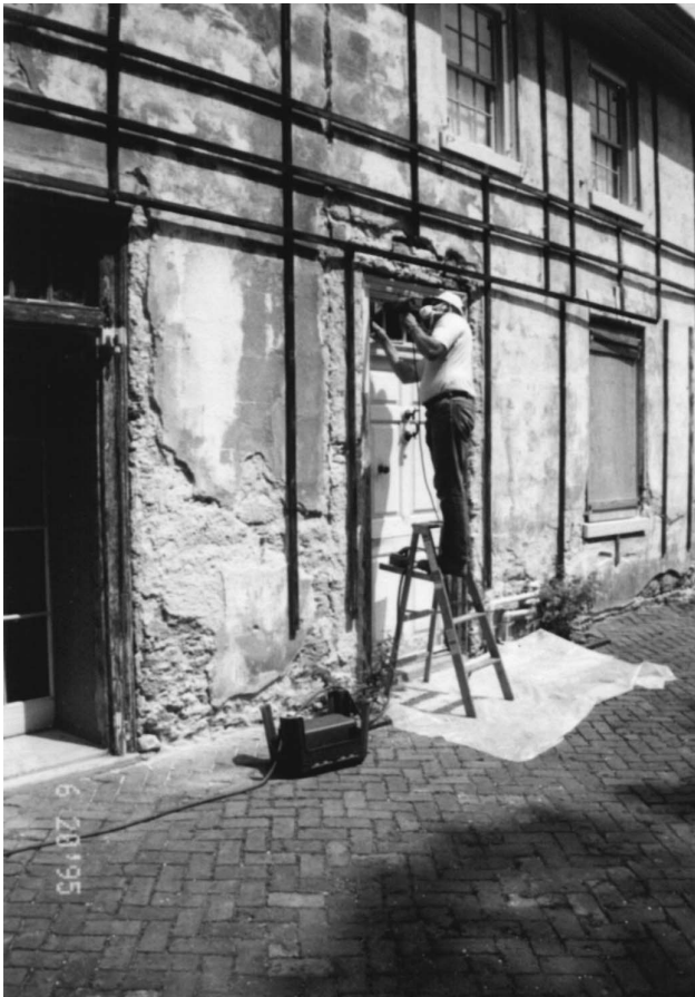
Removal of cement patches.
