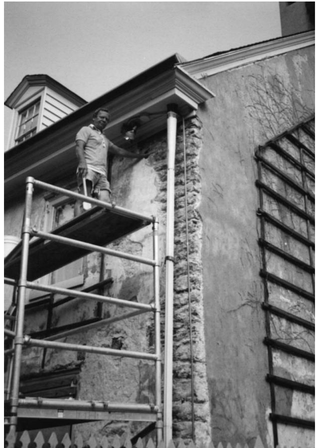
Joe Forrest cleaning masonry before stucco was applied.
