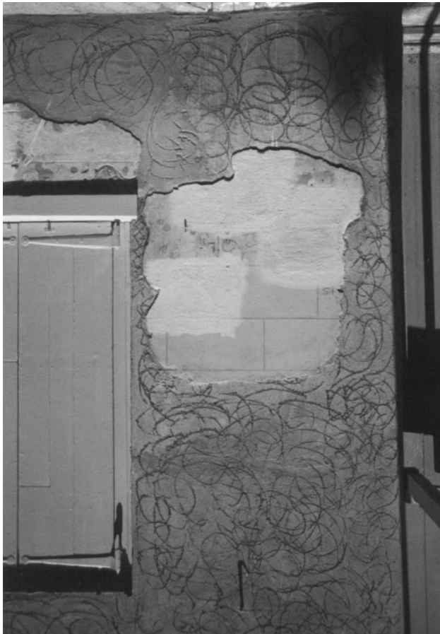
Building up stucco layers.
